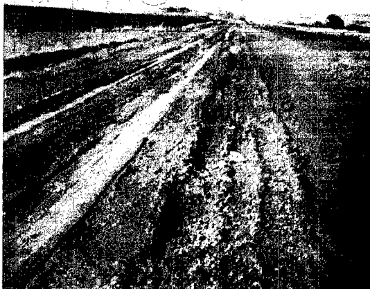
Persons living off main highways or ungraveled roads had their problems during the recent rainy spell. This heavily-traveled stretch of old Highway 35, a mile north of Hesking, was a typical problem-maker, with travel limited to four-wheel-drive vehicles until the sun finally came out and dried out the road enough to enable traffic to move normally again. The picture here was taken looking north.
